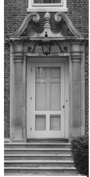
A good example of a sensitively designed storm door.
