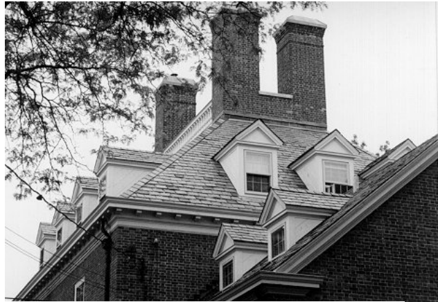
Extremely well maintained slate roof.
