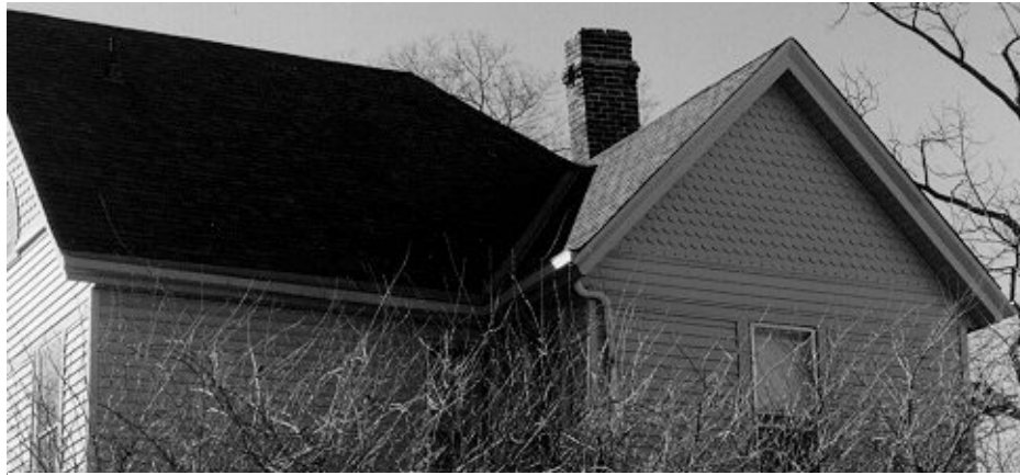
Pitched residential roof.
