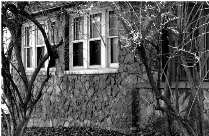
Good example of stone masonry.
