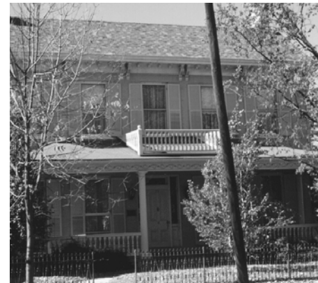
Wrought iron fence with a nice pedestrian path leading to the main building.
