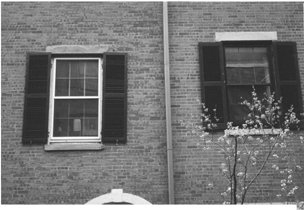
A coat of matching paint on a storm window and proper lintel maintenance can make the difference between a well maintained (right) and a poorly maintained (left) window opening.
