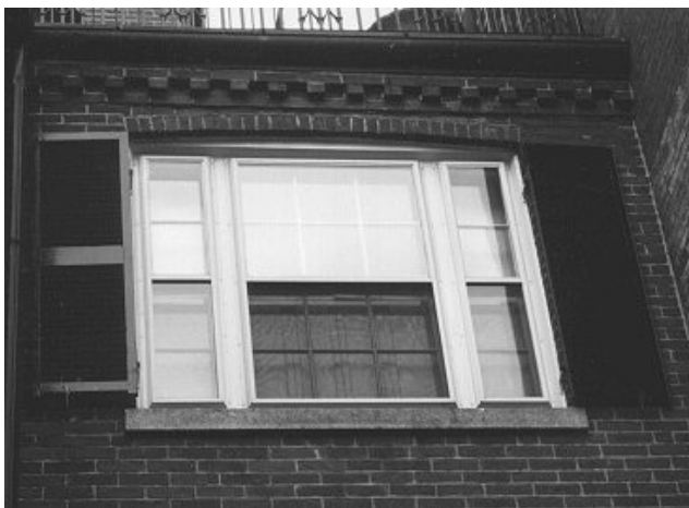
Clearly, these shutters could not cover the window opening and are thus inappropriate.
